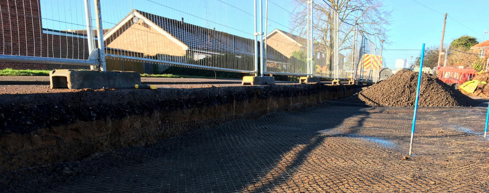
TriAx geogrid mitigated the risk of differential settlement and eliminated the need to import fill to provide a stable founding layers.
