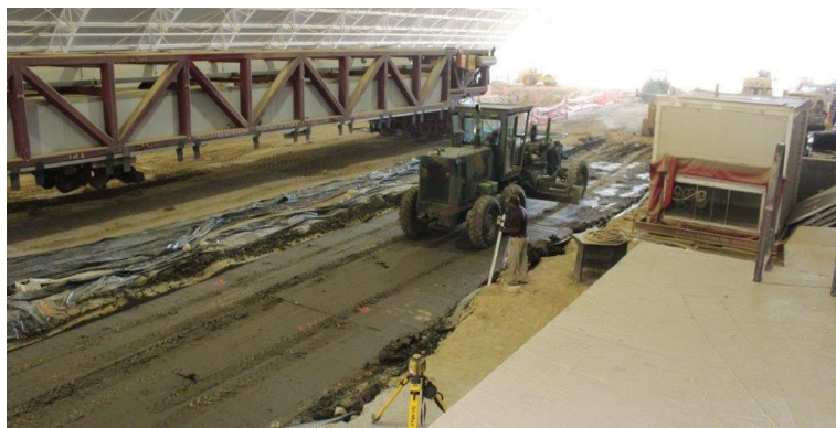
Figure 2 – Subgrade under construction at ERDC
